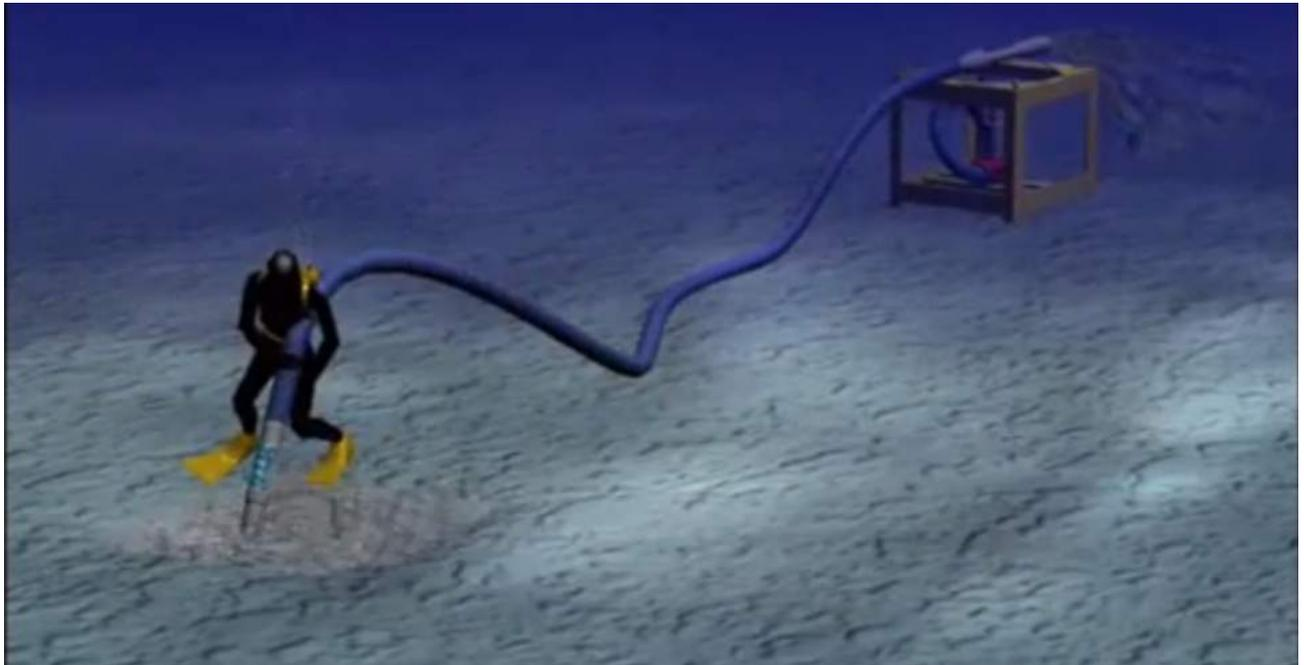
*Figure 6-189 Excavation Operation with Airlift (SediCon AS 2017)*
