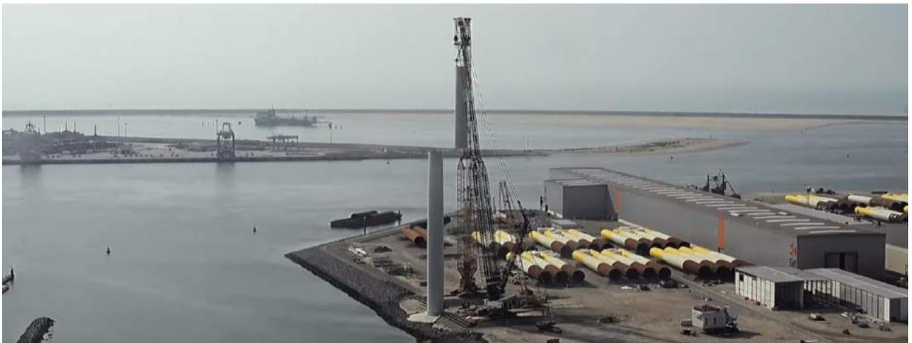
*Figure 6-16 Installation of the Fourth Segment of 12 MW GE X-Heliade WT in the Rotterdam Port (GE Renewable Energy 2019)*
