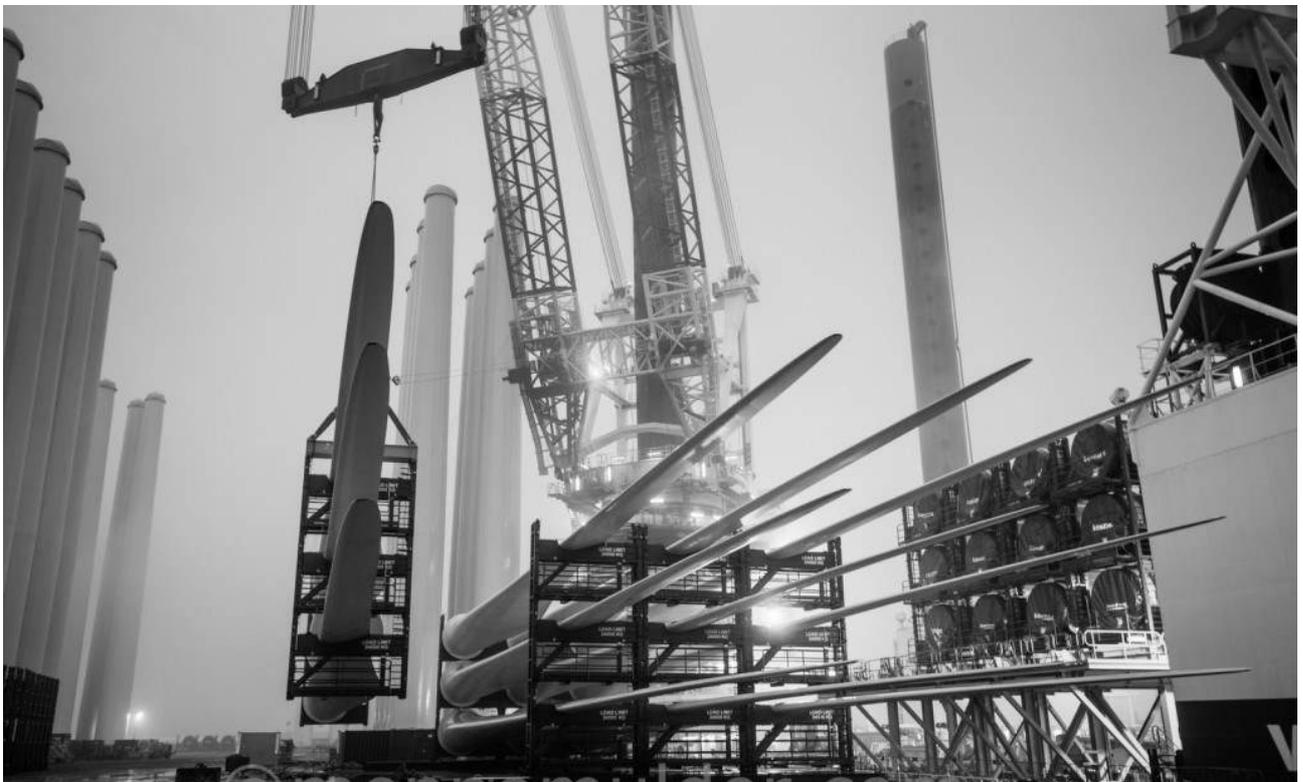
*Figure 6-58 Lifting Rack of Blades*
