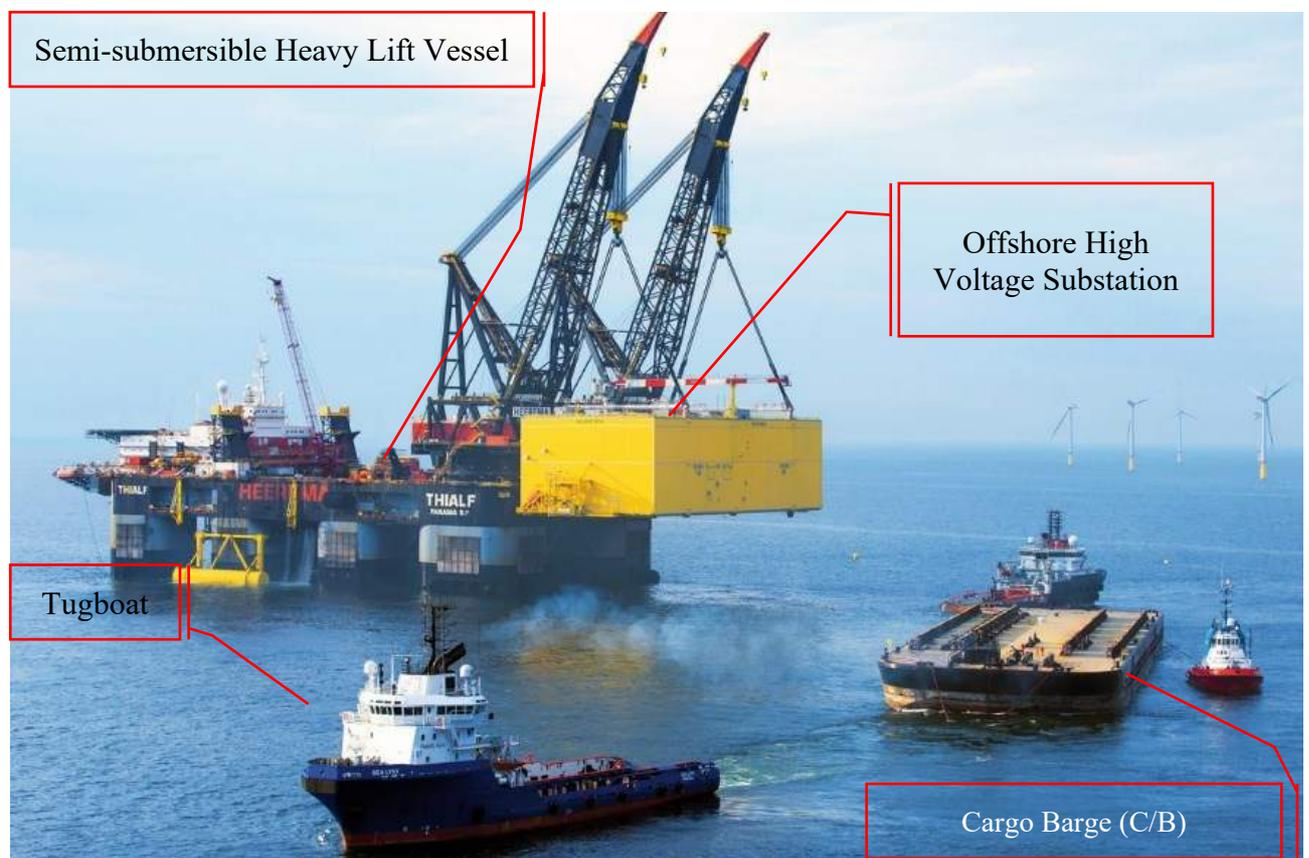
Figure 3-27 Installation of Topside of OHVS
