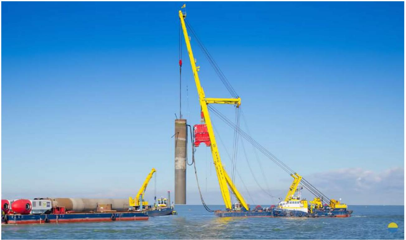
*Figure 6-117 Monopile is Extracted with Vibratory Hammer (Vattenfall 2016)*
