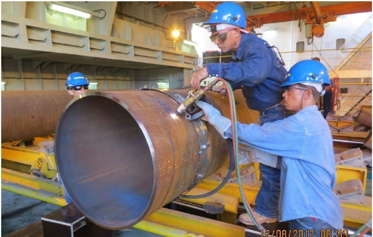
*Figure 6-143 Oxy Fuel Cutting Tools (Semi-Automatic)*
