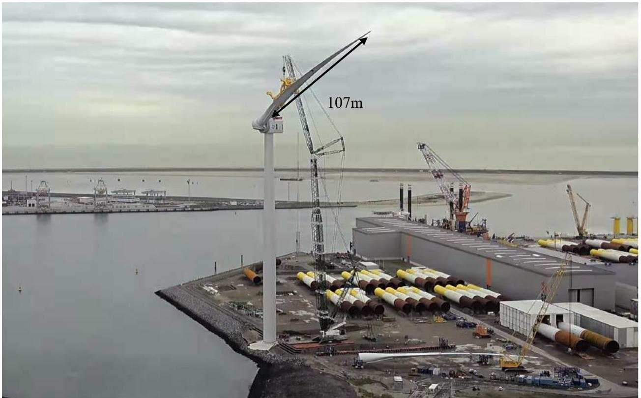
*Figure 6-18 Installation of First Blade of 12 MW GE X-Heliade Nacelle in the Rotterdam Port (GE Renewable Energy 2019)*
