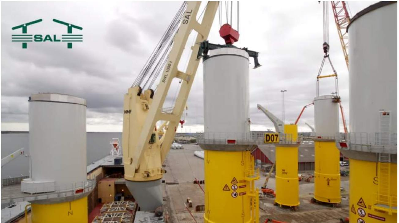
Figure 6-106 Lifting the TP with Hydraulic lifting Tool and Spreader Bar
