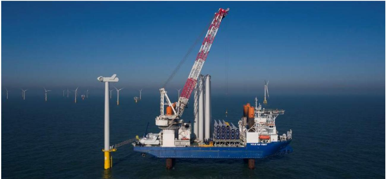
Figure 3-31 Installation of Nobelwind Farm by Vole au Vent Jack up Vessel (Jan De Nul Group 2017)
