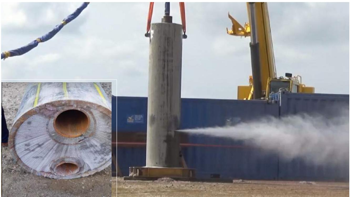
*Figure 6-3 Cutting of 36 inches Twin well Conductor*
