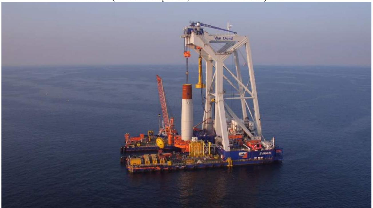
Figure 3-16 Feeder Configuration During Installation of Walney Extension (Van Oord 2017)
