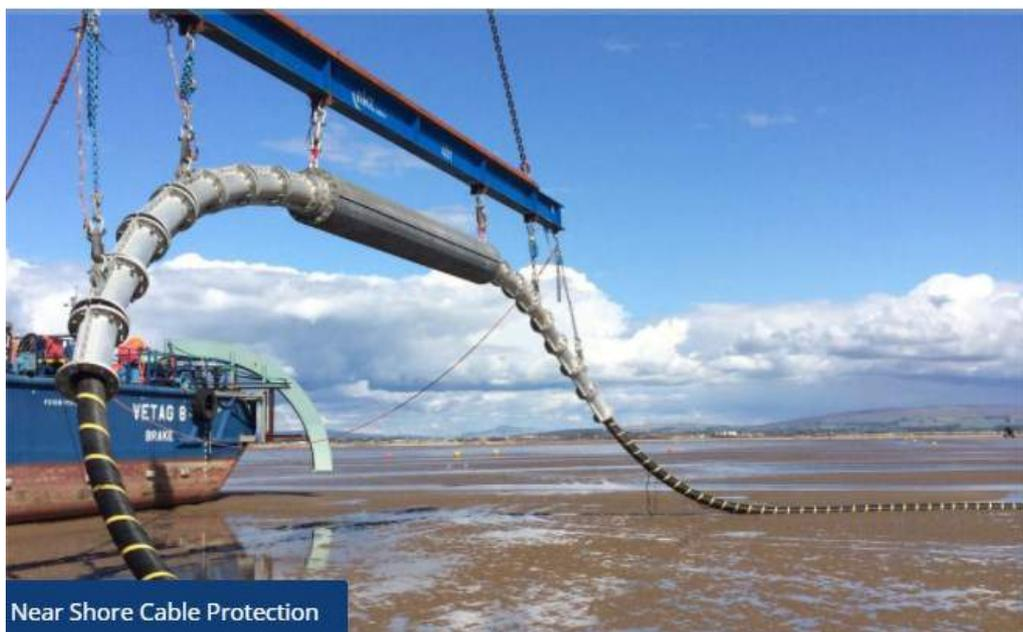
Figure 6-184 Near Shore Cable Protection (Tubular Protection) (TAGU OFFSHORE n.d.)
