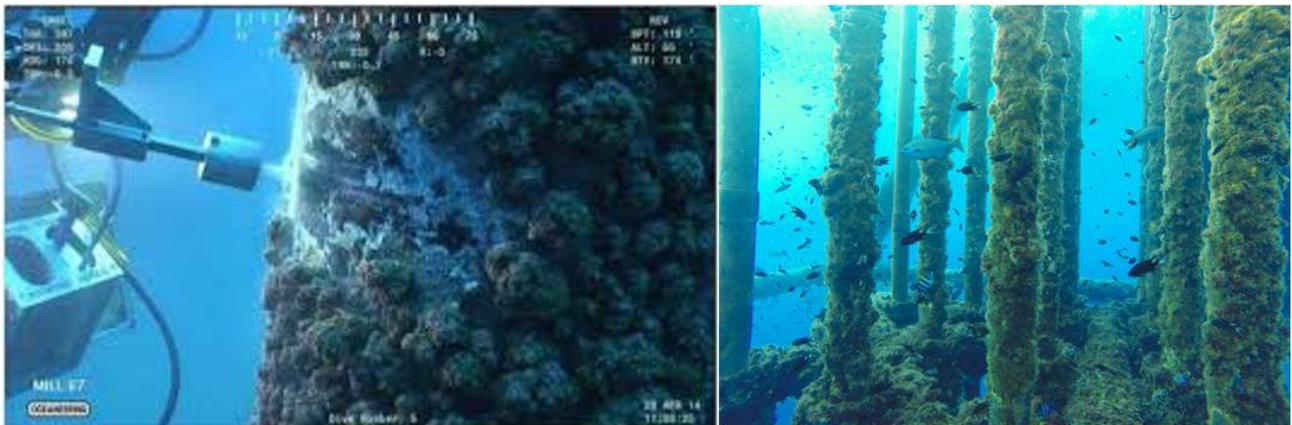
*Figure 6-155 Marine Growth attached to the Structure (Adobe Stock n.d.)*
