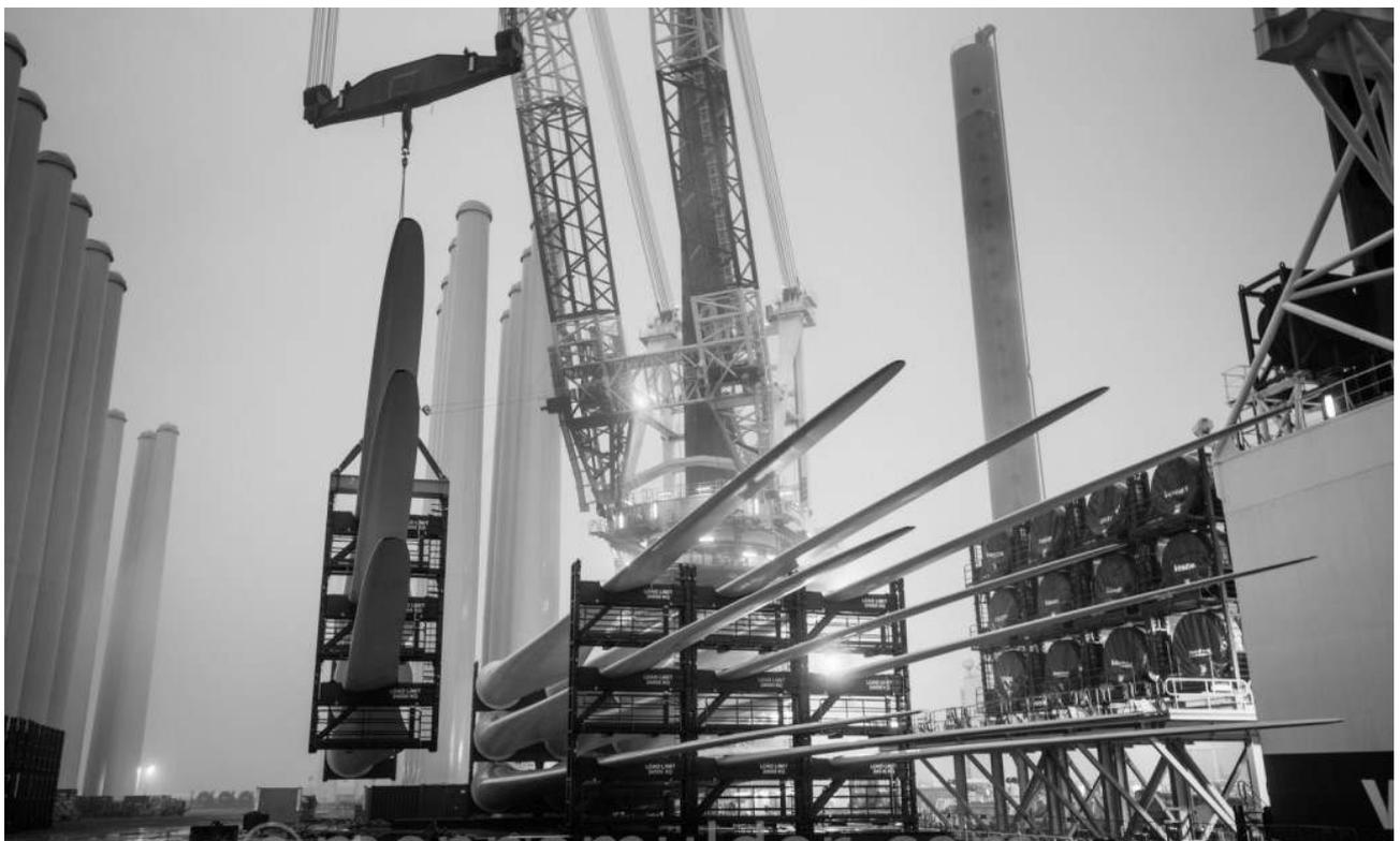
*Figure 6-58 Lifting Rack of Blades*
