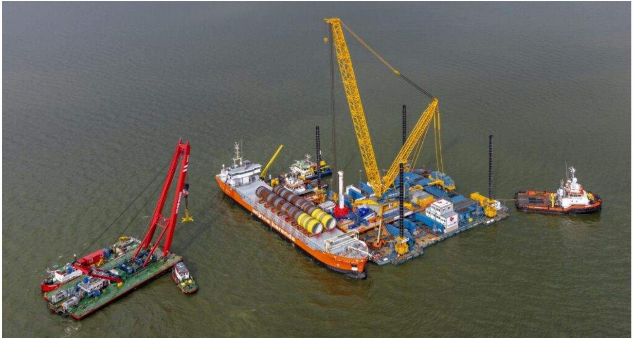
Figure 3-26 Installation of Frylan OWF in Feeder Configuration
