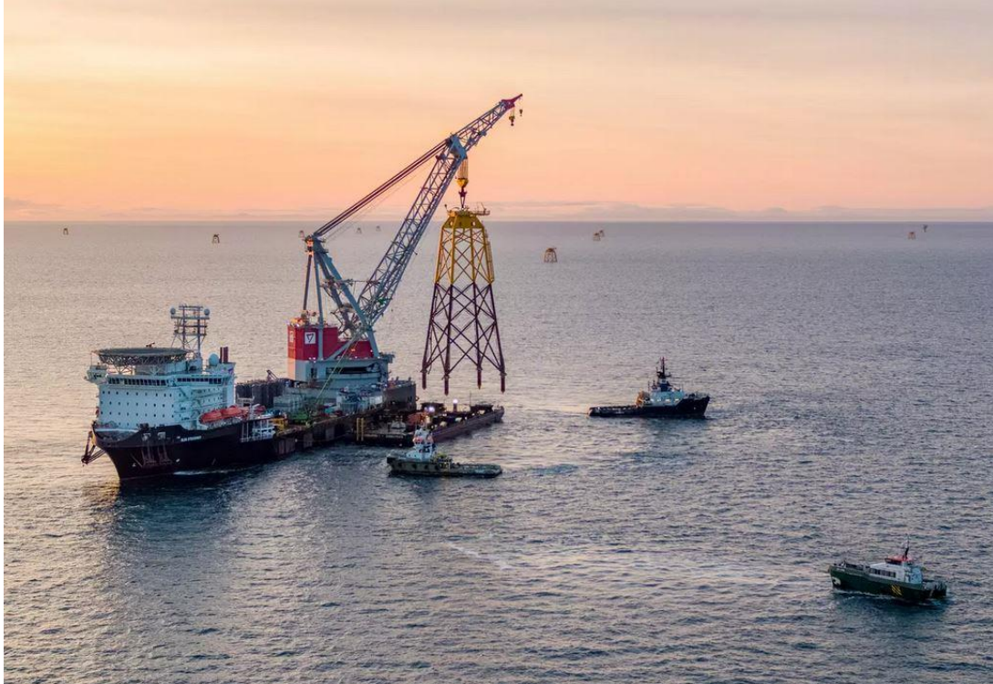
Fig. 1. Jacket installation for WTs in Beatrice OWF, UK 1
