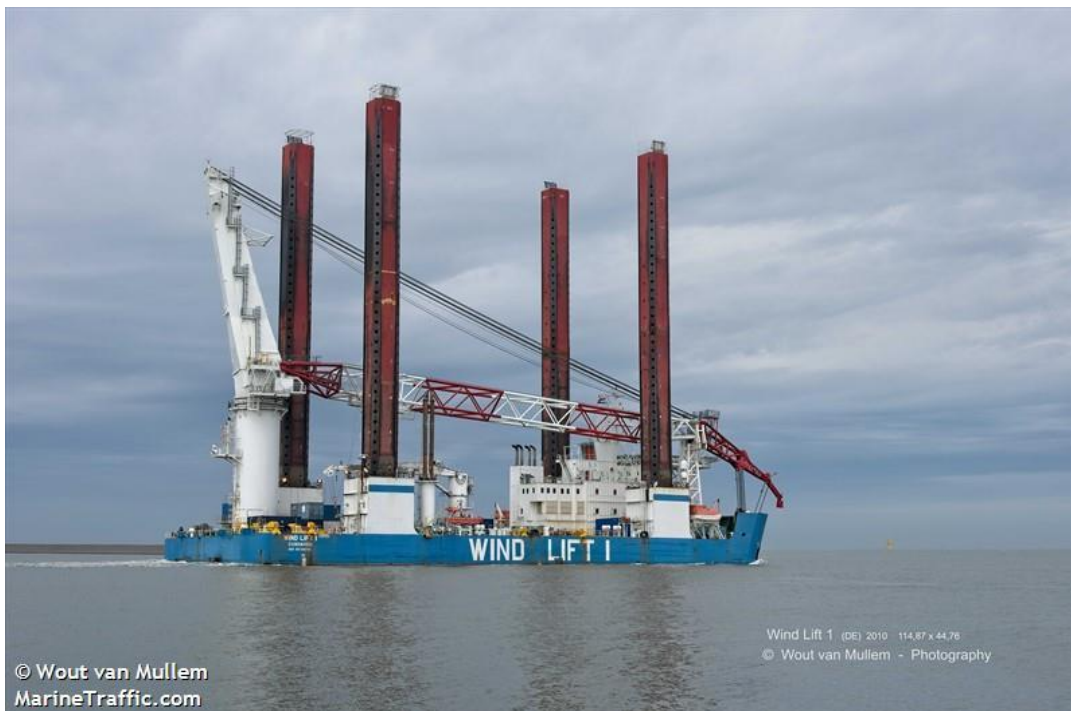
Fig. 10. Wind Lift I self-propelled JUV used for foundation installation in BARD Offshore I OWF
