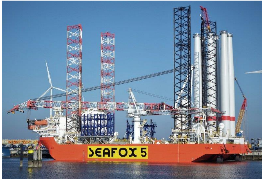
Fig. 9. Seafox 5 self-propelled JUV applied for foundation installation in Dan Tysk OWF 1
